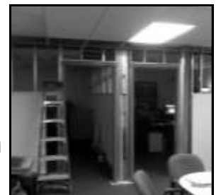
HALF WALLS TO FULL WALLS AND DOORS
